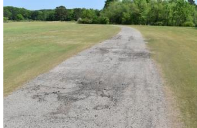
Browns Mill cart path renovation
