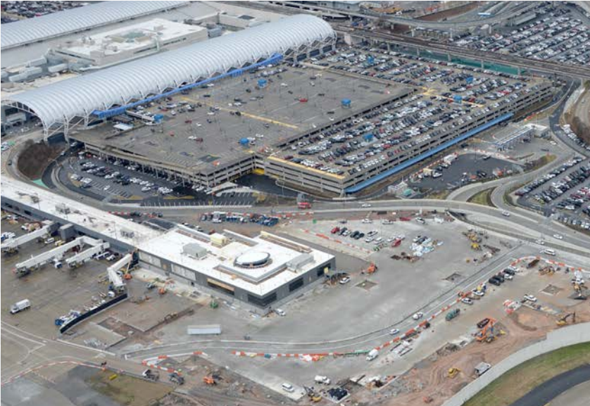
CONCOURSE T-NORTH EXTENSION ($158M) COMPLETION: DECEMBER 2022
