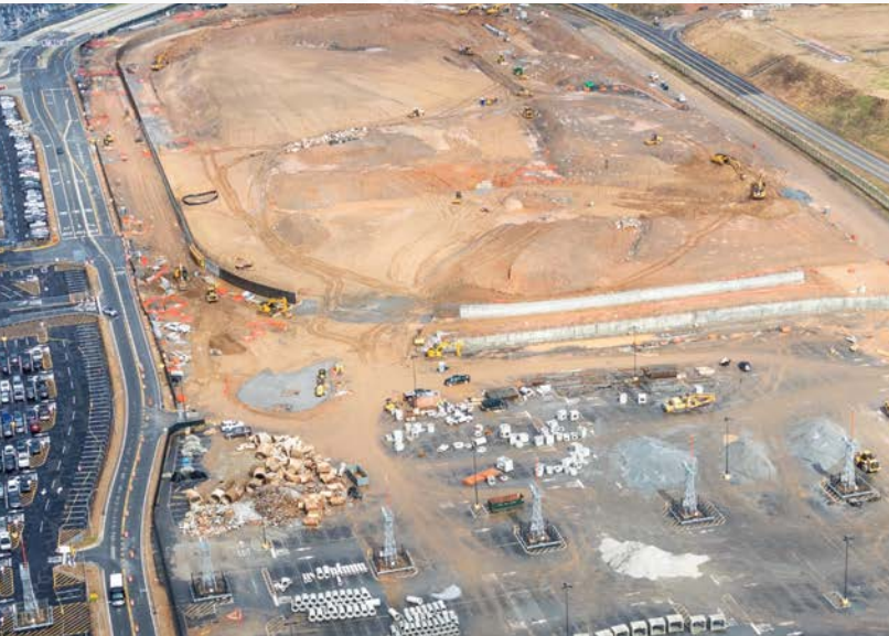
RUNWAY 9L END AROUND TAXIWAY ($62M) COMPLETION: DECEMBER 2022
