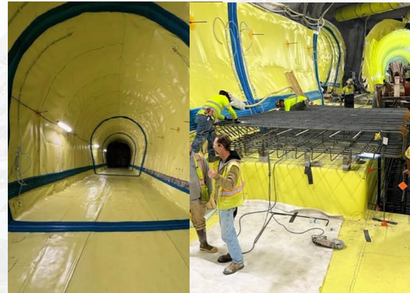
PLANE TRAIN TUNNEL EXTENSION COMPLETION: FEBRUARY 2024
