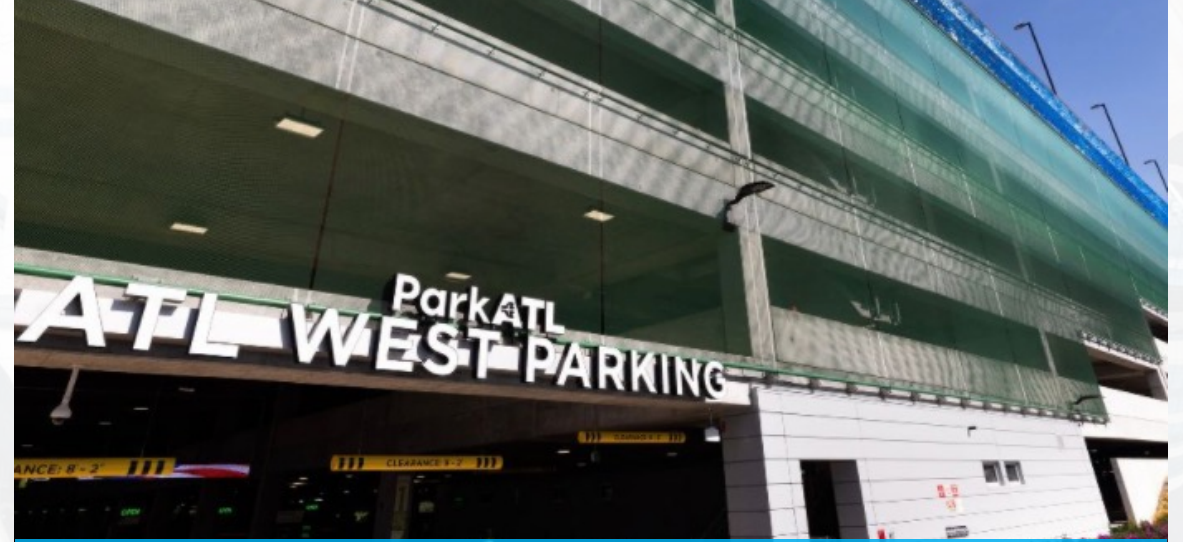
ATL WEST PARKING DECK MAIN ENTRY WAY
