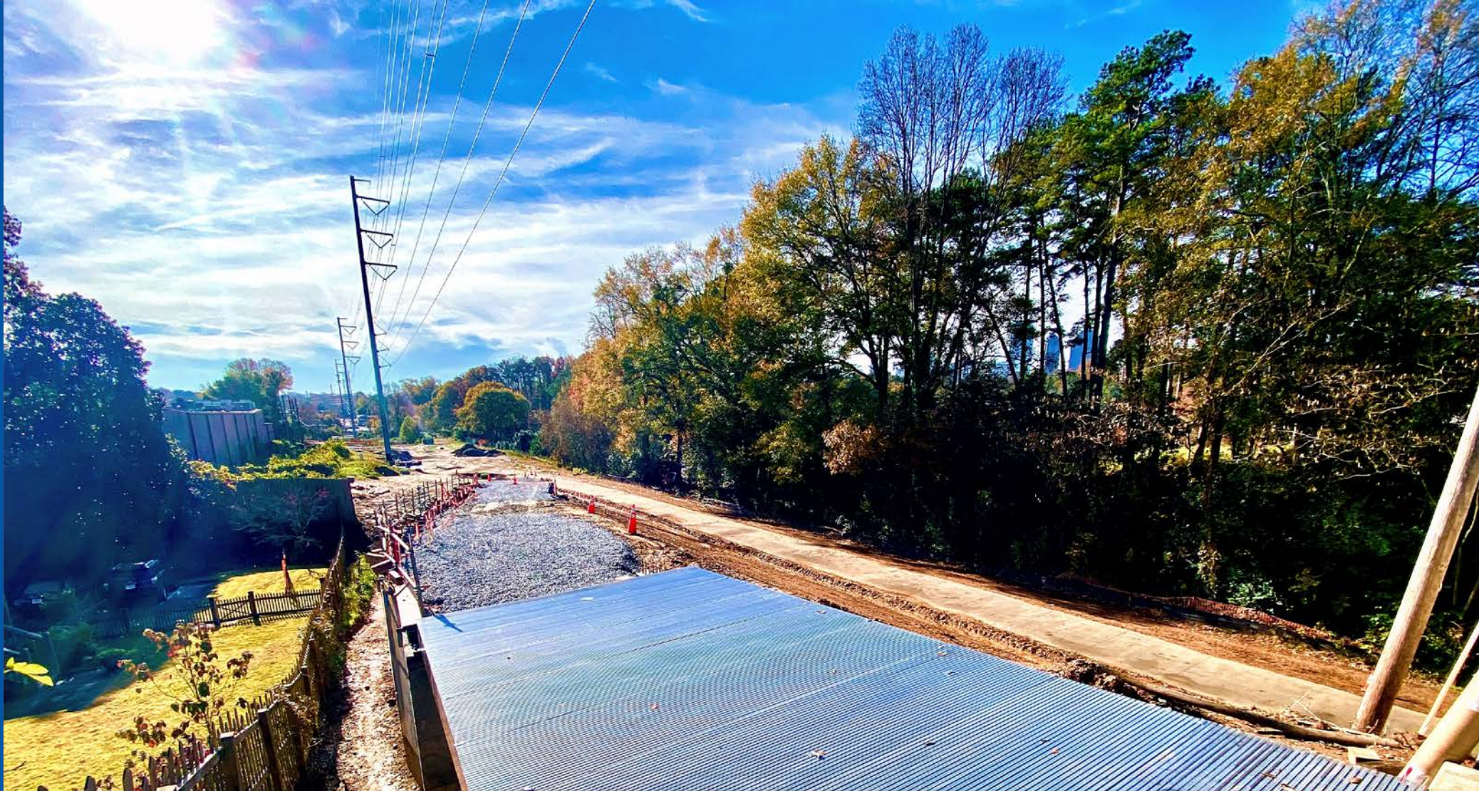
Interim Northeast Trail Construction Montgomery Ferry Ramp November 2020
