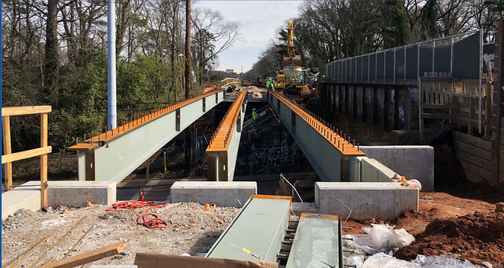
Southside Trail West Construction Metropolitan Parkway February 2021
