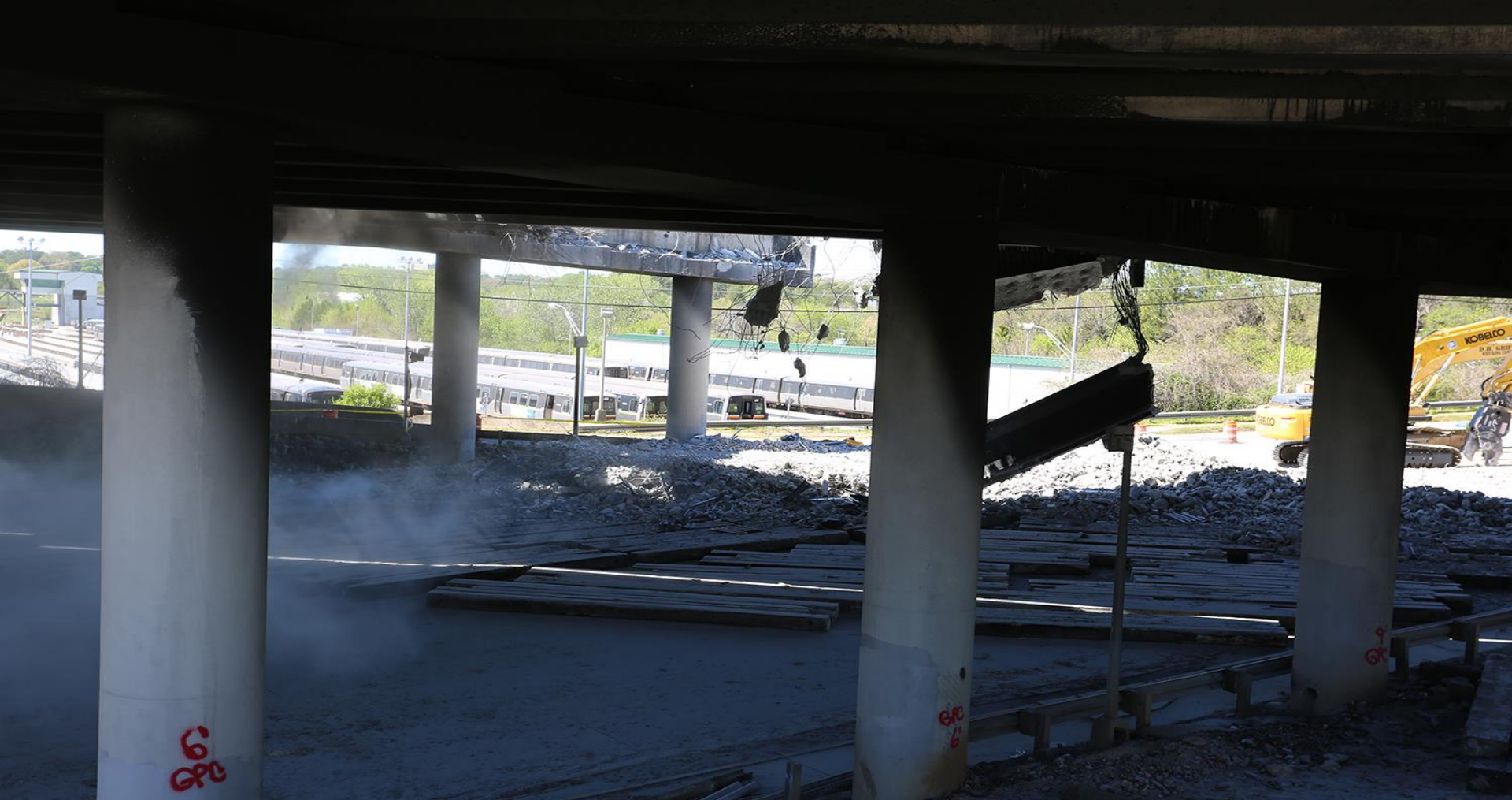
Removal of Span over Piedmont Road
