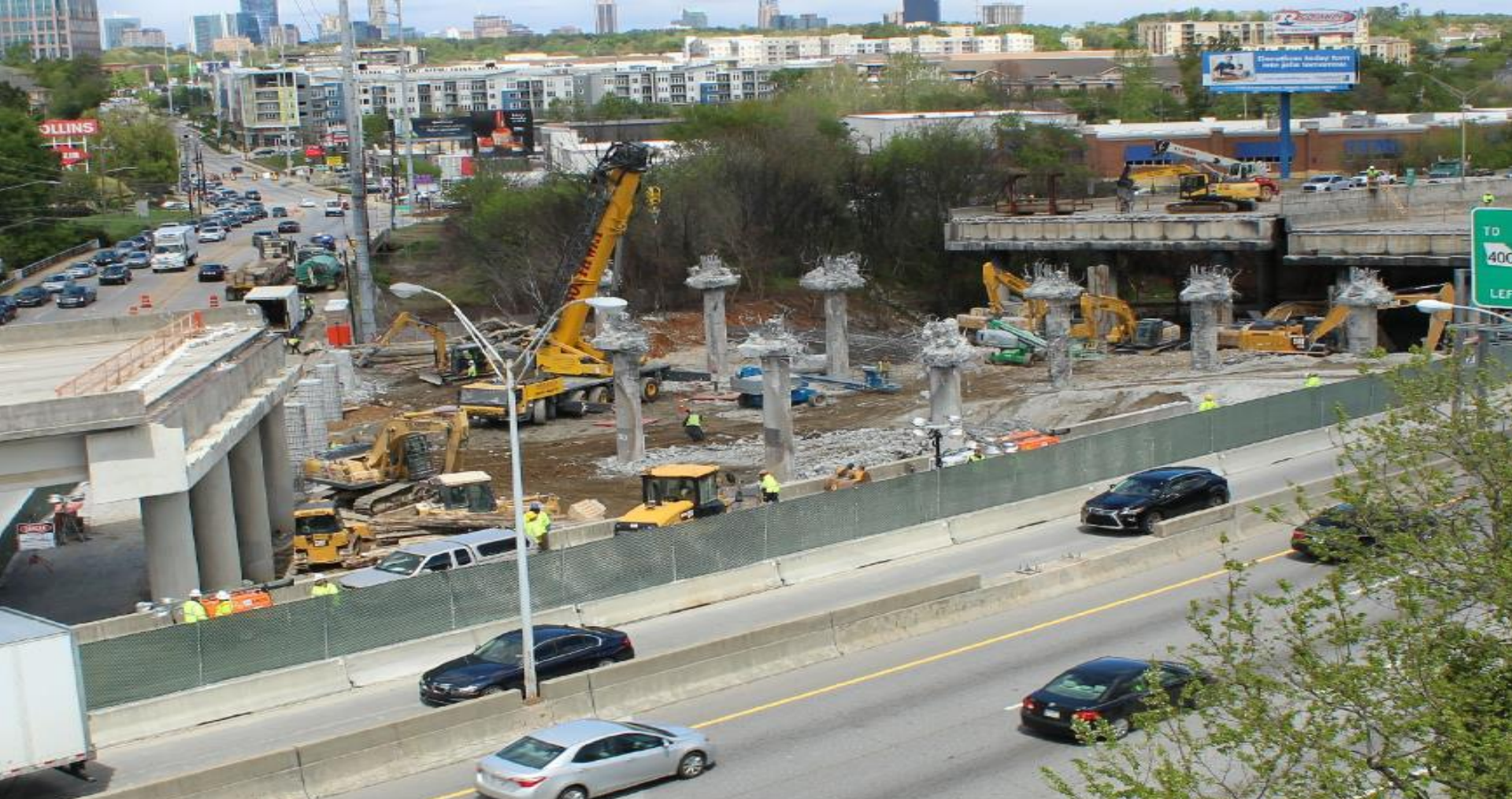
Interstate 85 Bridge Rebuild – Thursday afternoon, April 6, 2017
