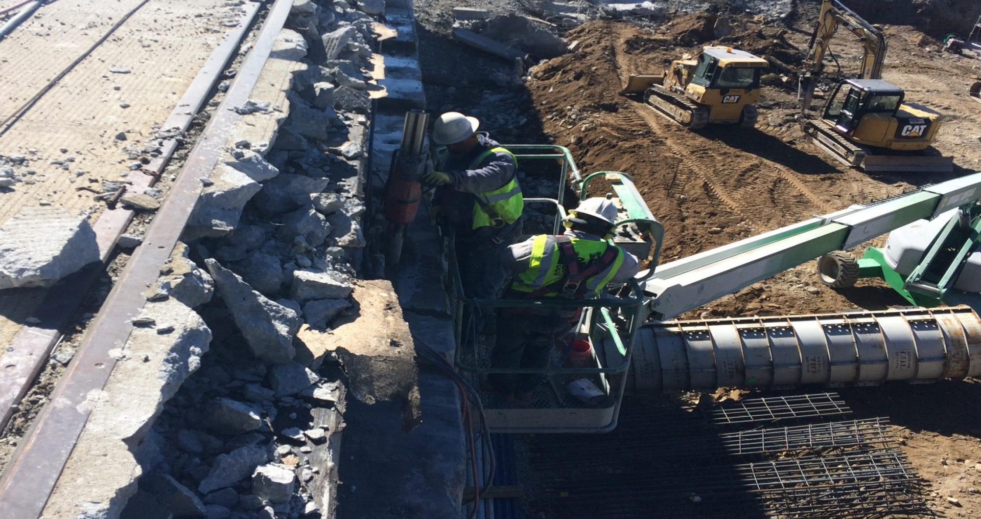
Removal of Existing Dowels
