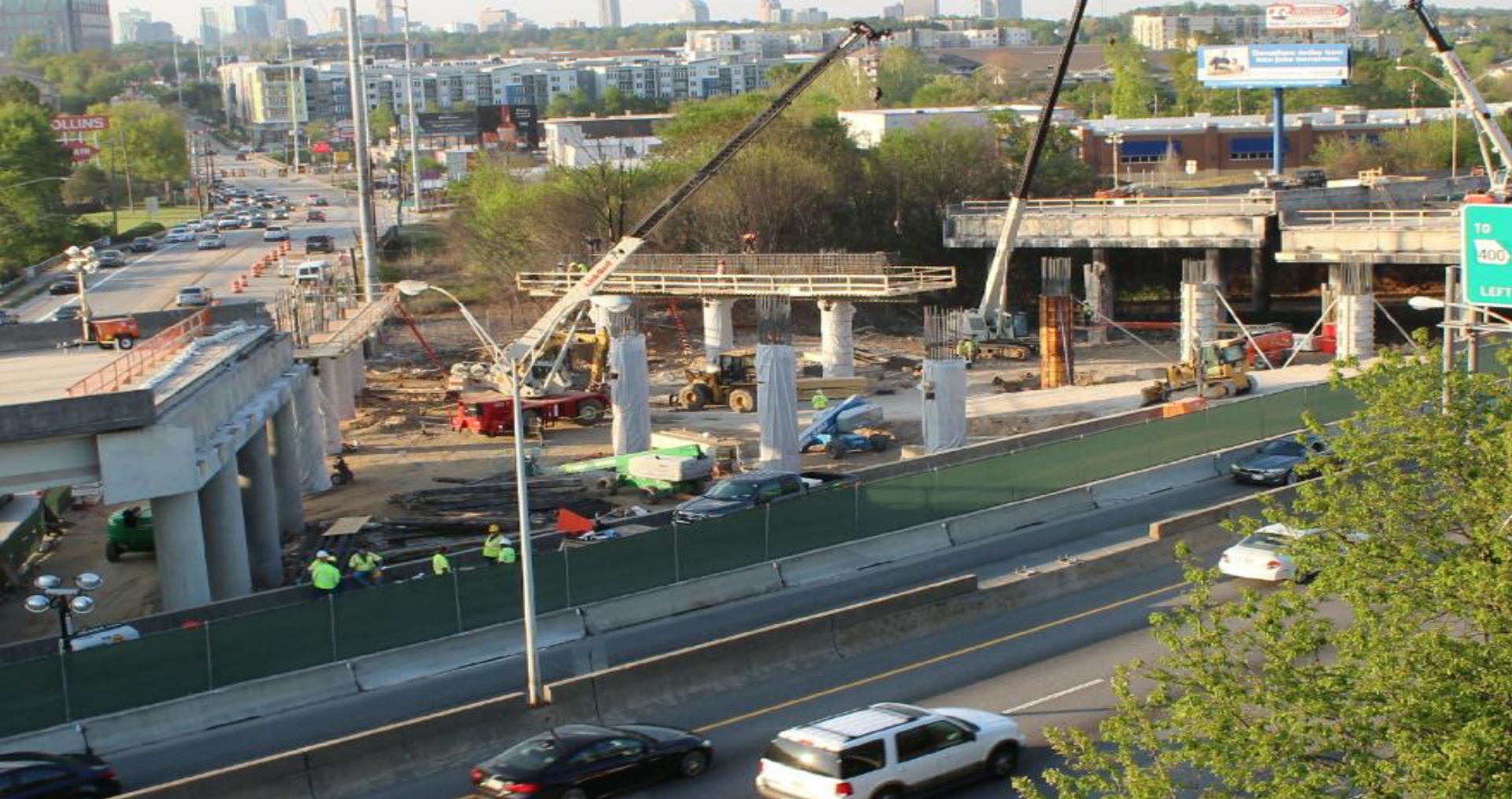
Interstate 85 Bridge Rebuild – Tuesday afternoon, April 11, 2017
