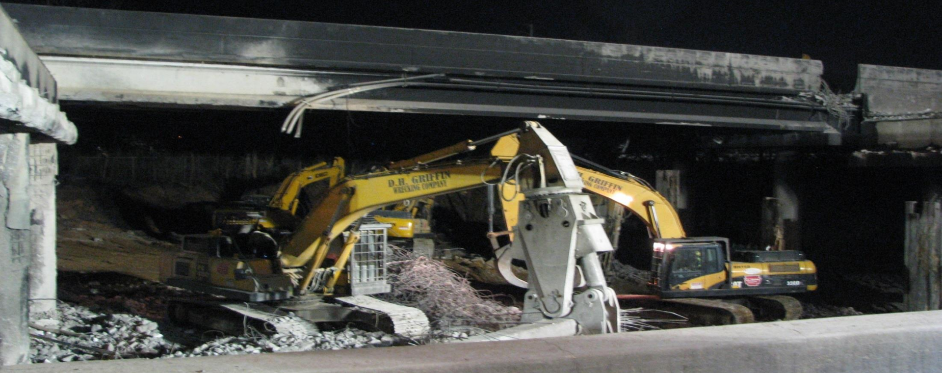
Demolition of Collapsed Span - March 31, 2017
