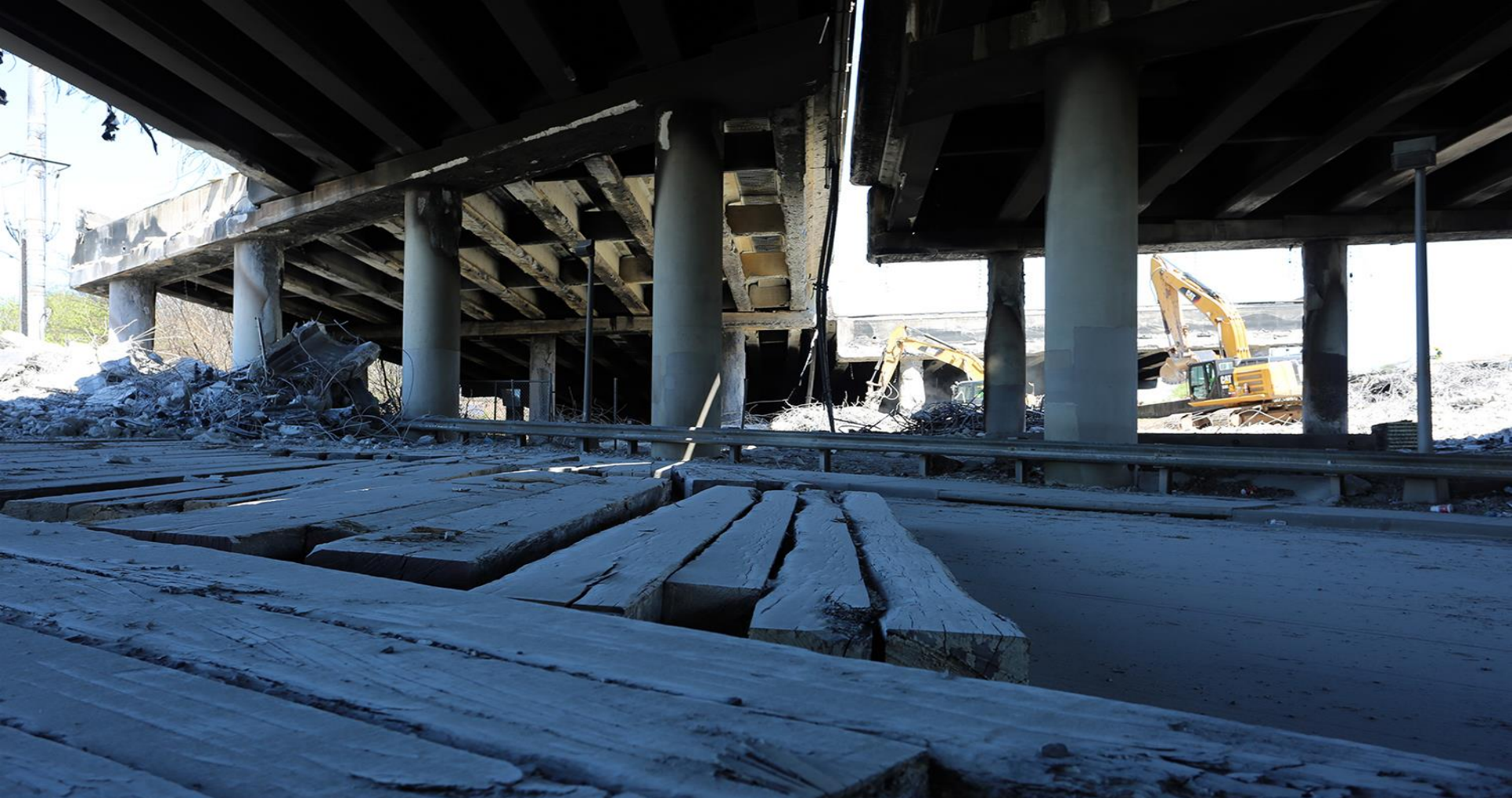
Removal of Span over Piedmont Road
