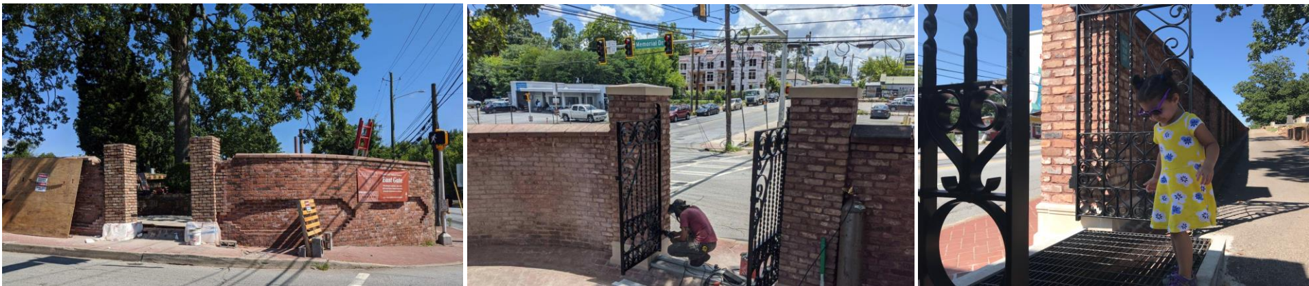
Historic Oakland Foundation, Eastside
