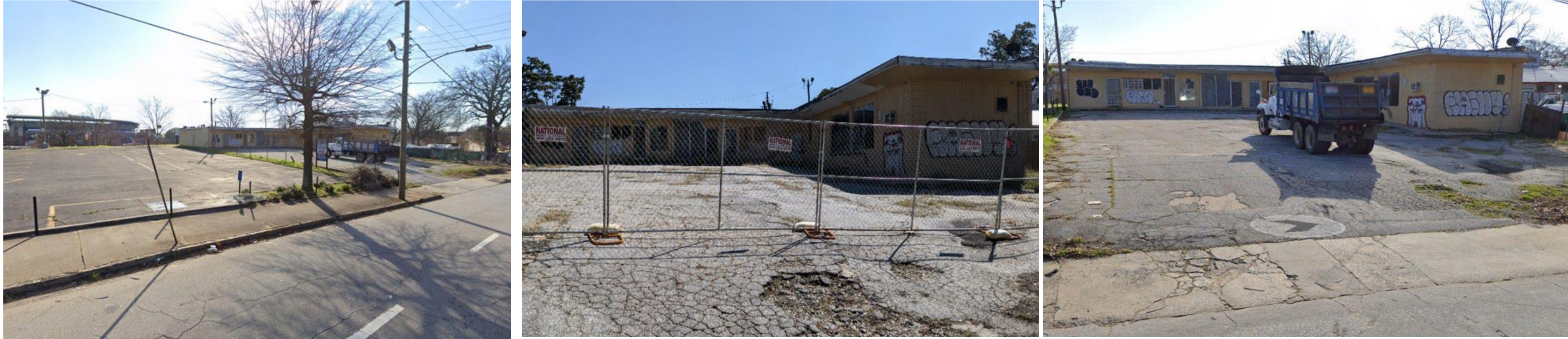
Hunter Pryor Street Enterprises – Small Business Improvement, Stadium Neighborhoods
