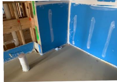
Exterior - taping of seams (Tyvek weather wrap. Placement of Ardex, bathrooms
