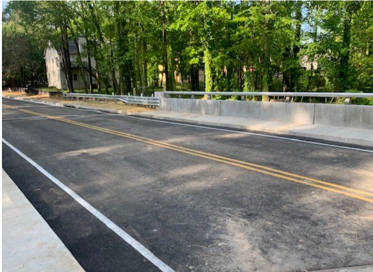
Childress Drive Bridge
