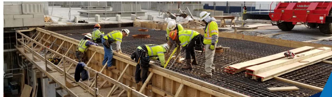
Construction underway on the Spring Street Viaduct
