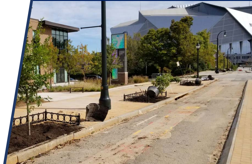
North MLK Drive SW, and Walnut Street SW
