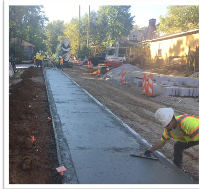
Sidewalk installation underway on the Hirsch Street roadway improvements project
