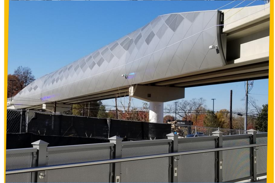
Northside Drive Pedestrian Bridge
