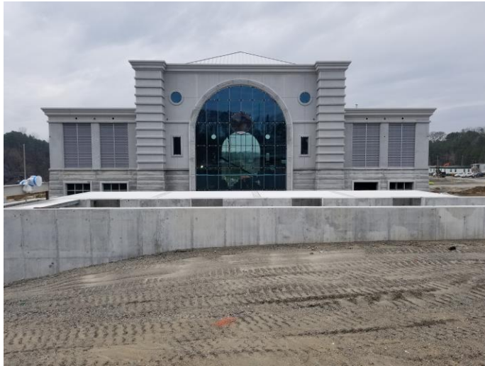
Quarry Pump Station – East Elevation
