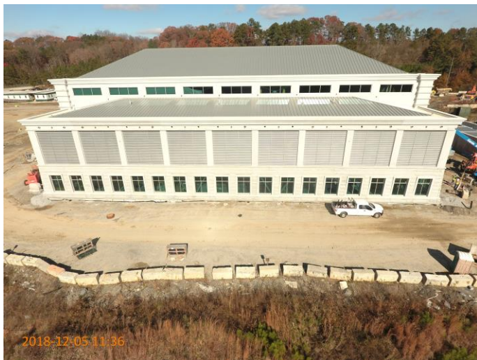
Quarry Pump Station – South Elevation
