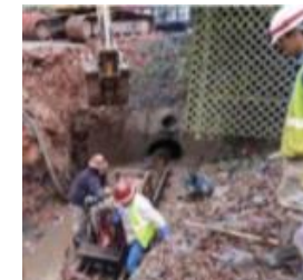
483 Monument Avenue SW
