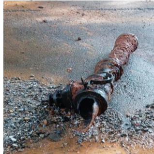
Fire Hydrant Service Repair
