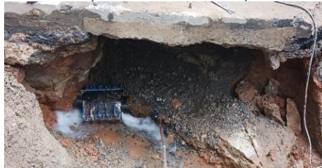
Damaged Sleeve
