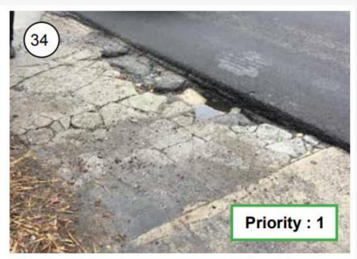
Issue: Cracked sidewalk; no curb between sidewalk and roadway
