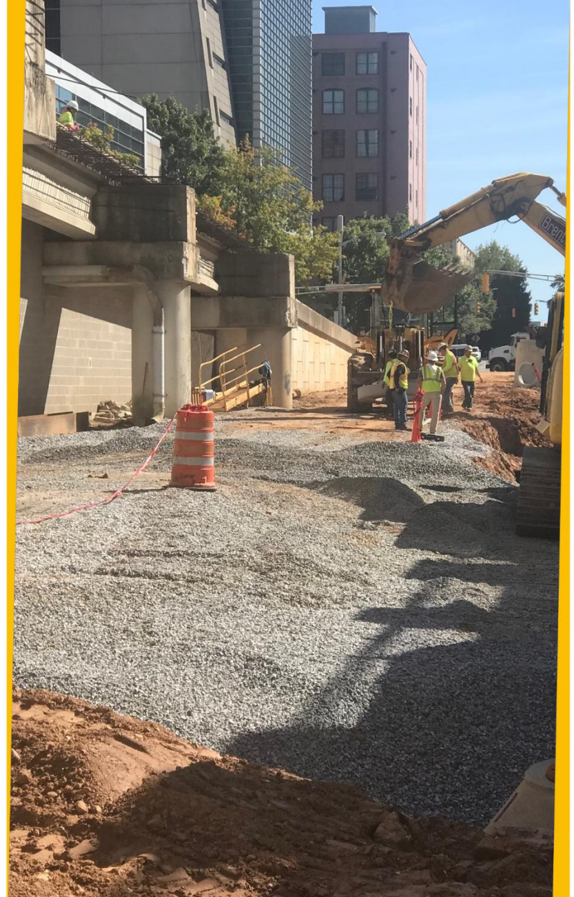
Spring St. Bridge
