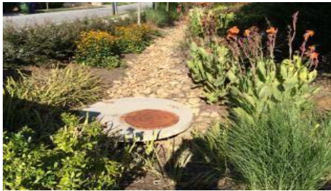
Bioswale - Edgewood Townhomes
