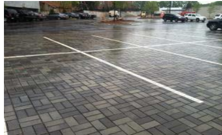
Permeable Pavers - Urban Market on Howell Mill
