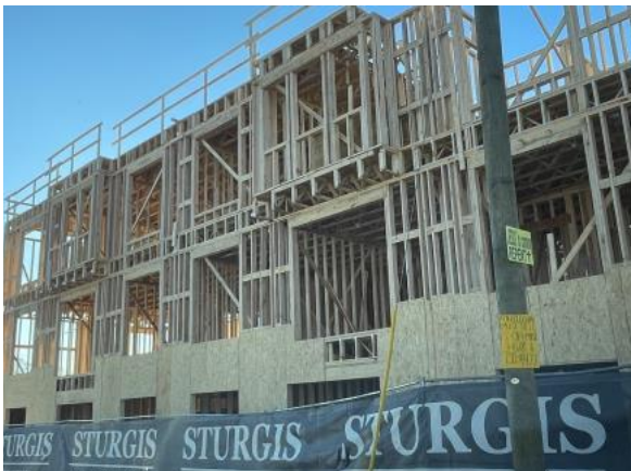
Abbington at Ormewood 42 Affordable Units | $16,588,853 TDC
