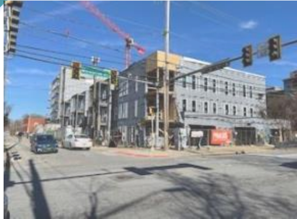
Madison Reynoldstown 116 Affordable Units | $33,295,000 TDC
