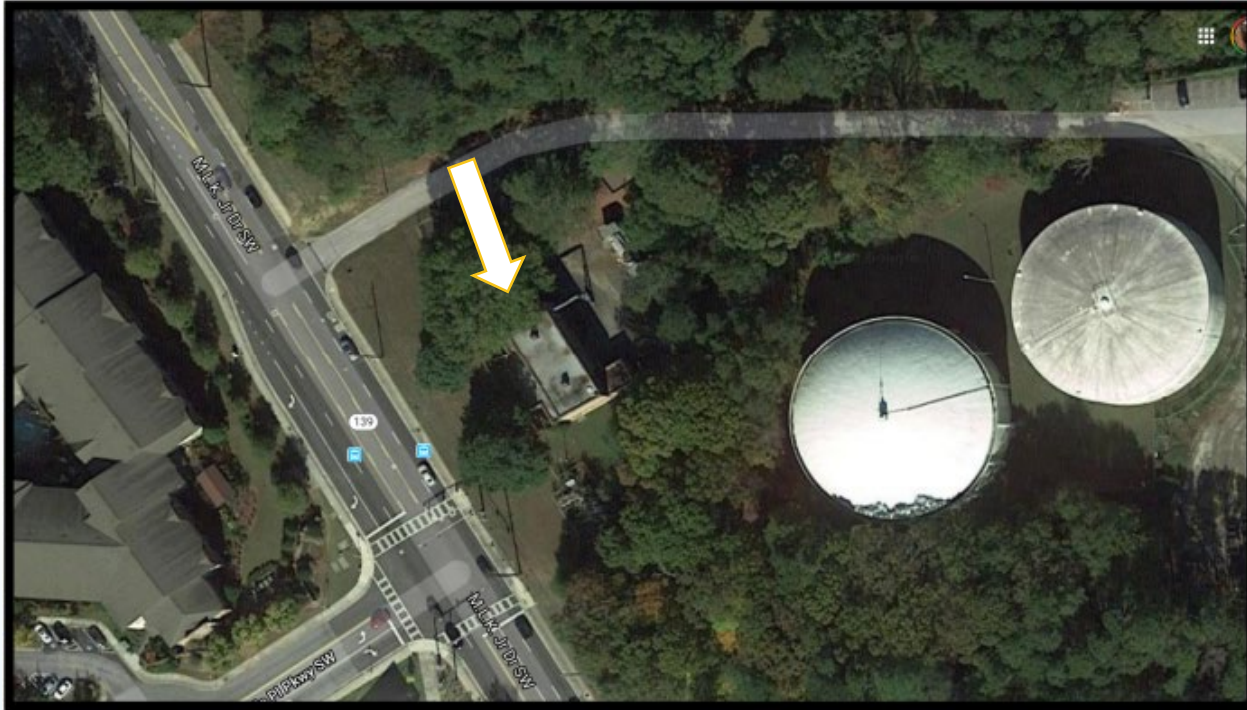
Adamsville Pump Station - Highlighting Project Location
