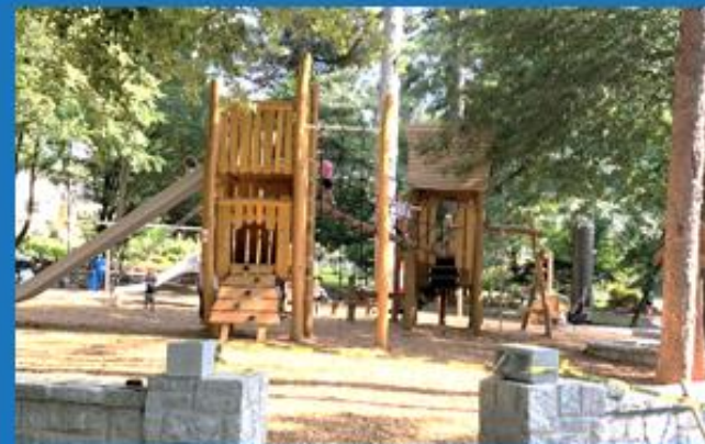
Playgrounds at Noble Park & Sara J. Gonzalez Park in Progress
