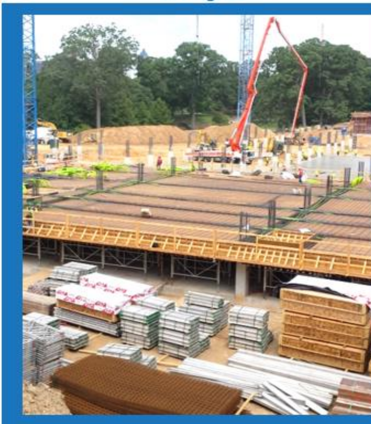
Grant Park Gateway in Progress
