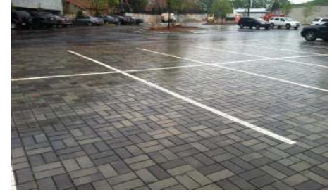
Permeable Pavers - Urban Market on Howell Mill
