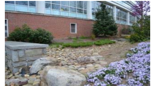
Bioswale – GT Klaus Building
