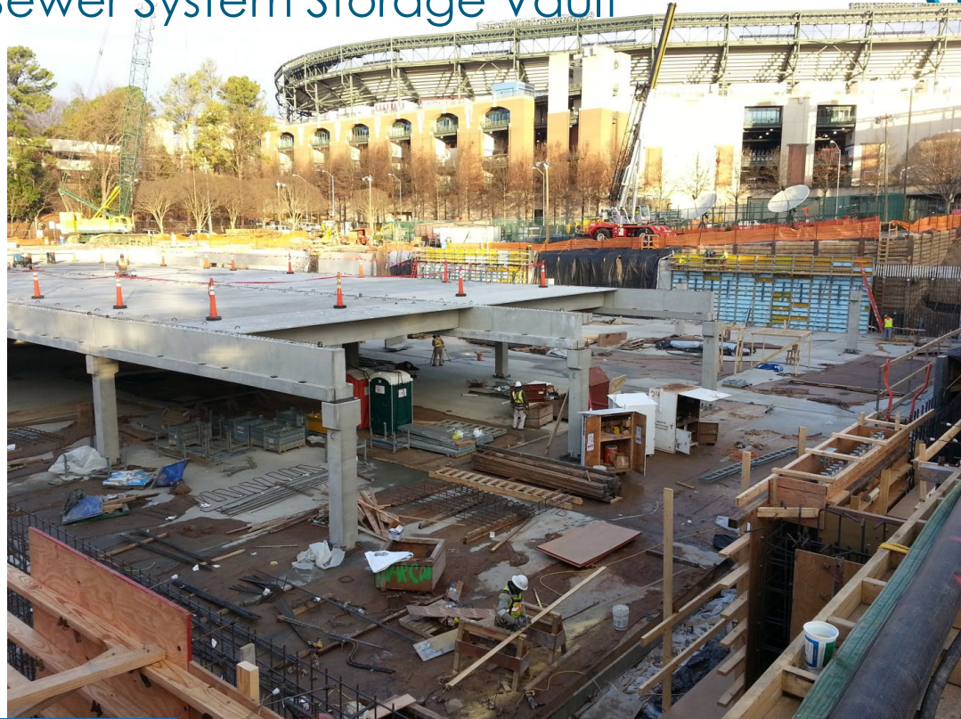
Construction – Media Lot Vault 5.9 MG
