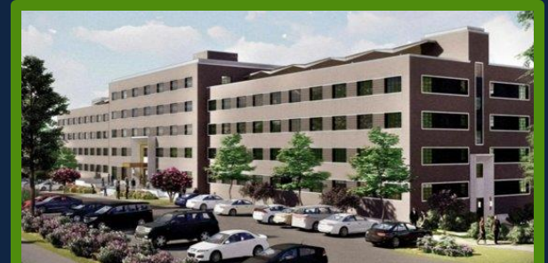
Heritage at Westlake is projected to house 102 PSH tenants when the project is completed in the coming years.
