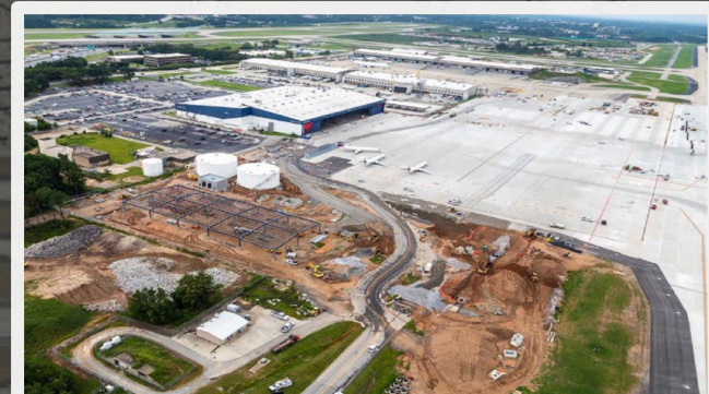
South Deicing Complex | $165.7M
