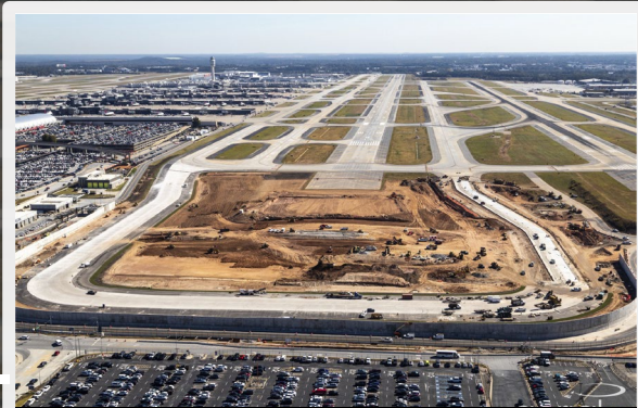
Runway 9L End-Around Taxiway | $64.9M
