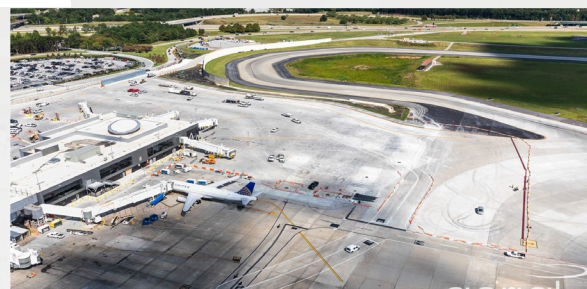
Concourse T-North 5-Gate Extension | $317M
