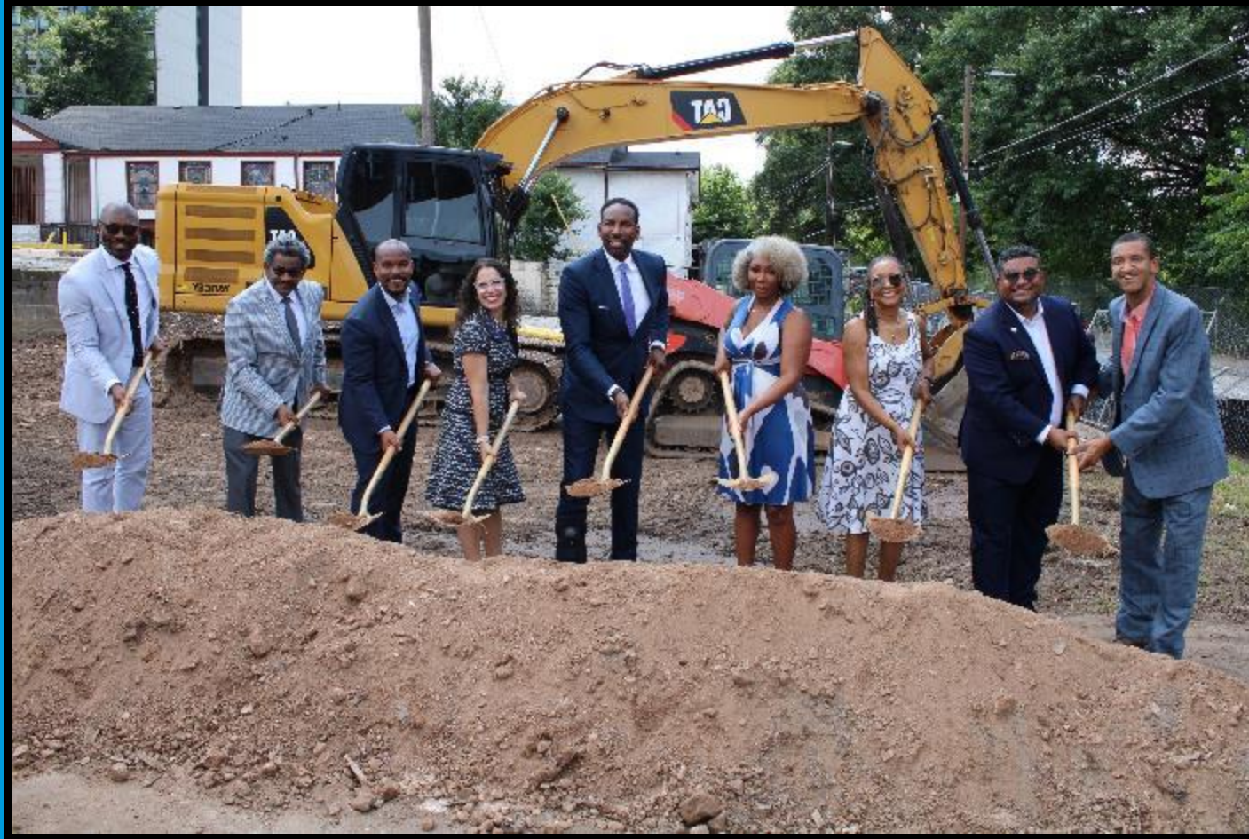
Front Porch Sweet Auburn Groundbreaking $3 M Eastside TAD grant, $11 M AEMI allocation
