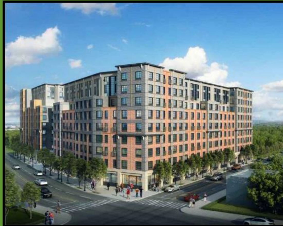
1090 Hank Aaron Drive: 250 units of affordable housing at 60% AMI or below
