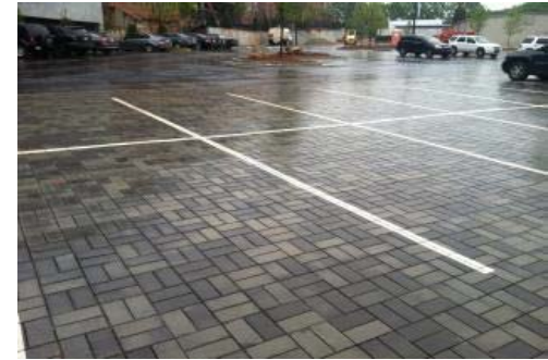
Permeable Pavers - Urban Market on Howell Mill
