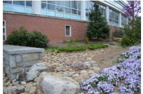
Bioswale – GT Klaus Building
