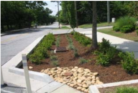
Stormwater Planter - Whitehall Terrace SW
