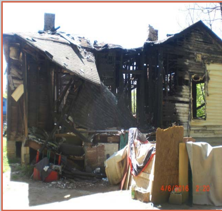
Demolition Project Before
